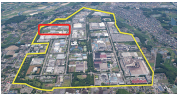
New plant at Kiyohara Industrial Park for Utsunomiya Kiki Co., Ltd. (photo care of Tochigi Promotion Council of Establishment of New Business Facilities)
