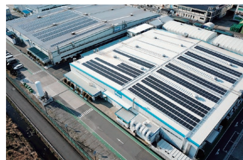
Solar power generation at Koyo Machine Industries Co., Ltd.'s Yuzaki Plant
