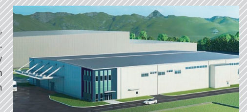
Image of a new plant for manufacturing lithium-ion capacitors upon completion
