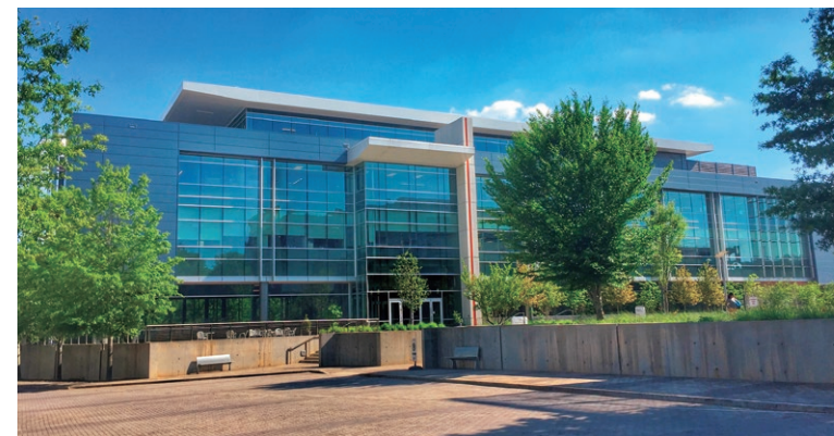
JTEKT North America Headquarters
