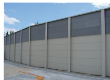
Sound barriers (Nara Plant)
