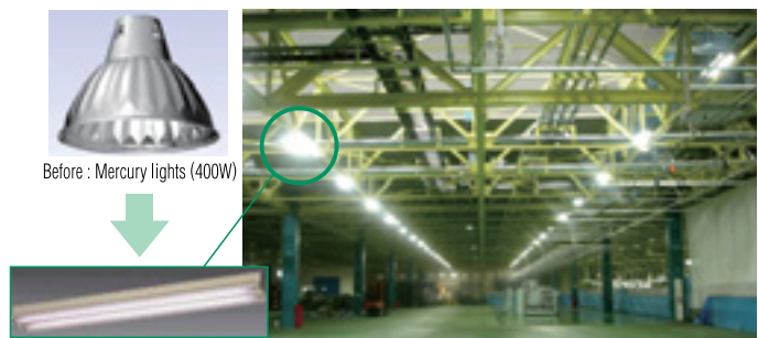
High-efficiency fluorescent lights (Four Hf 32W bulbs) [Kariya Plant / Higashi-Kariya Plant / Hanazono Plant]
