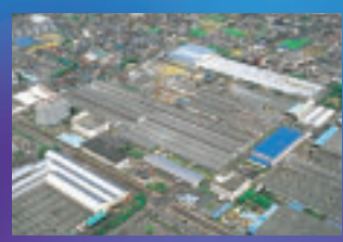
Head Office and Main Plant
