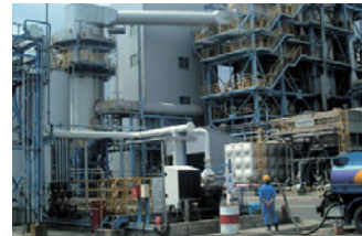
On-site check of incineration facility (July 2005)
