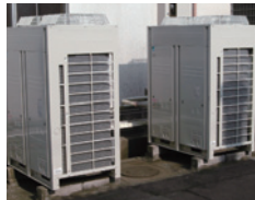
Replacing GHP with high-efficiency EHP
