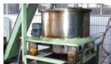
Collect oil using a centrifuge and reuse
