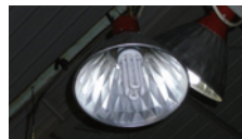
Conversion from mercury lamps into high illumination fluorescent light
