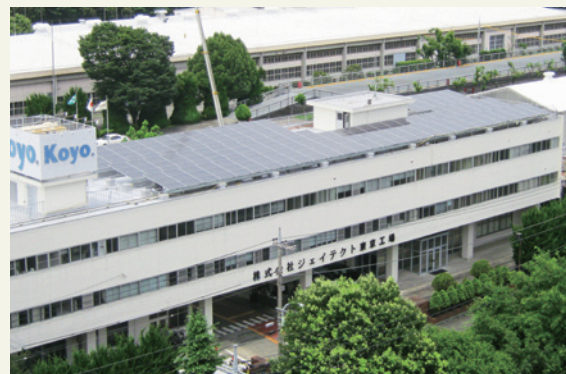
Solar power generation (Tokyo plant)
