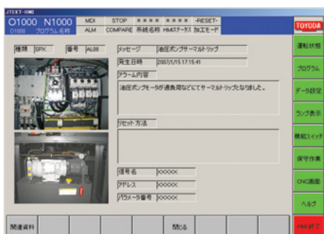
Fig. 4 Example of detailed alarm screen
