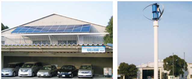
Kagawa plant (solar and wind power generation)
