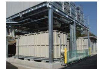
Photo of nighttime thermal storage air conditioning system: Thermal storage area is on the bottom and the heat pump is on top
