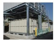
Photo of nighttime thermal storage air conditioning system: Thermal storage area is on the bottom and the heat pump is on top
