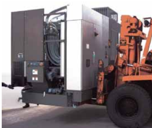
図 9 機械搬入 In the process of installation
