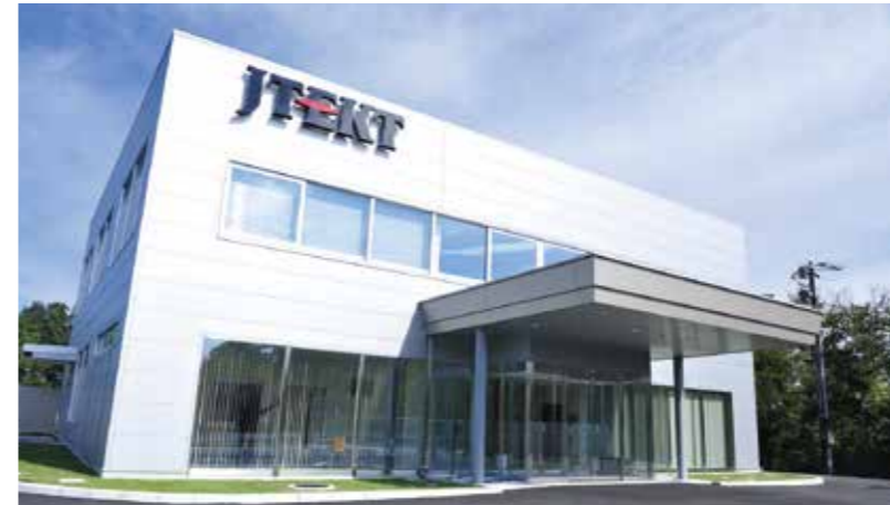
管理棟 Administration Building
